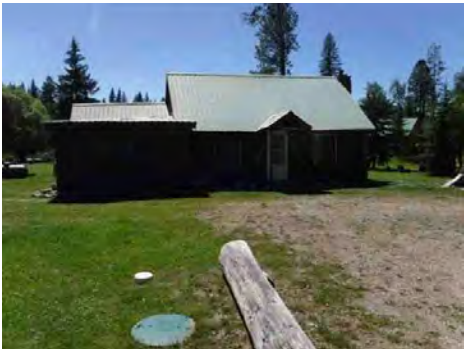
Front, Septic Location
