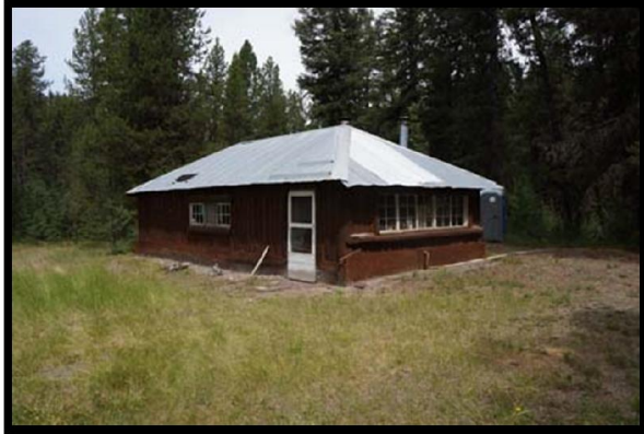
South and East Sides of Cabin
