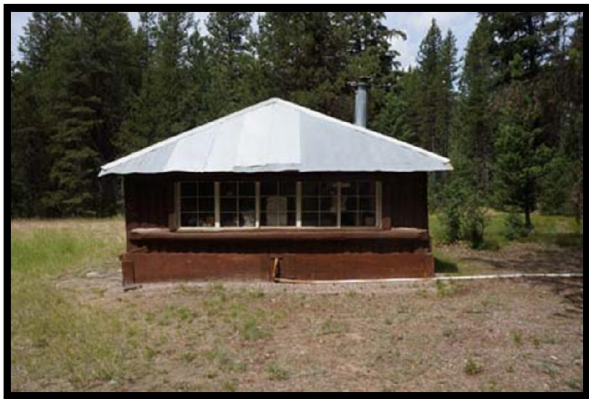
East Side of Cabin
